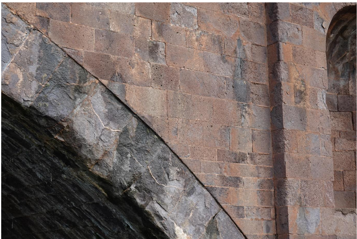
I believe the arch to be a veined Limestone. It doesn't seem to take well to runoff from the volcanic stone above which are the volcanic Trap, available from various quarries in the neighbourhood.
