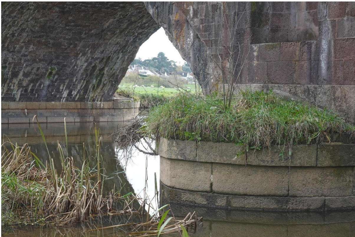
The vegetation on the northern cutwater is quite something. I suspect that the surface is flat enough for soil to deposit when the river is high. With the natural drawdown through the width, it is likely that the river covers this side when it doesn't cover the other.
