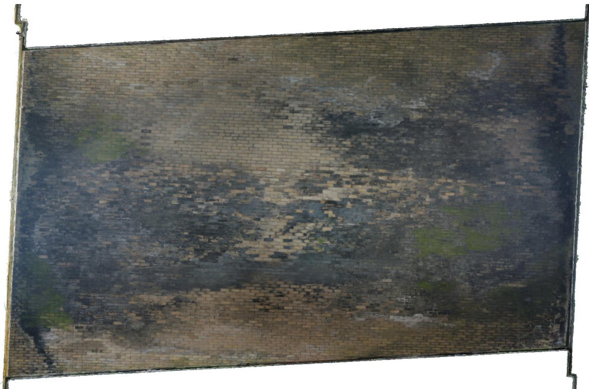
Figure 3 Soffit with 101 photos from SONY A7Rii
