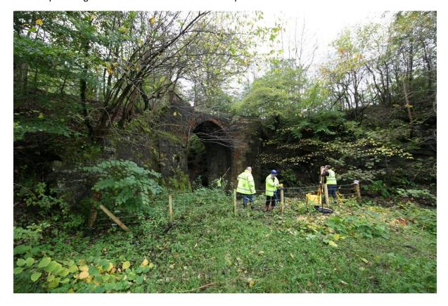
There is the cliff on the right and a rather high approach embankment on the left. The embankment was certainly just tipped and not compacted. If I remember rightly it was mostly ash.
