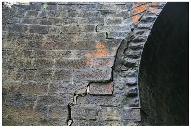
And further up the wing wall is pushing out past the edge of the arch. A look further back shows how that fits together with the rest of the wing wall and an added buttress.
