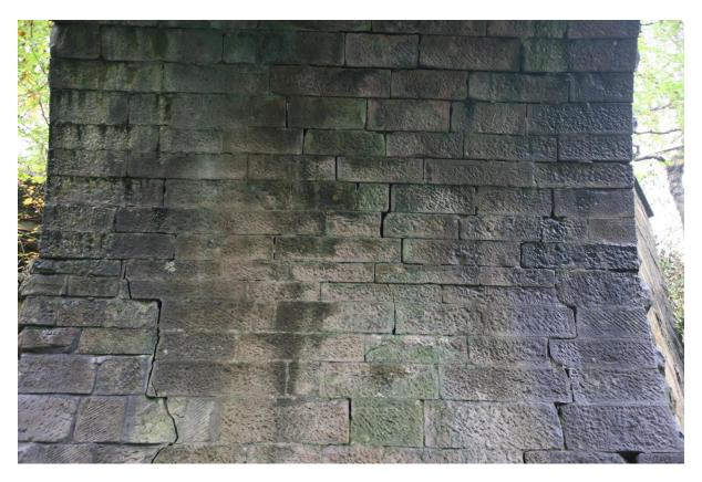
What's going on here? The beds don't come near to matching to the left of the left hand crack. Has that bit been rebuilt?
