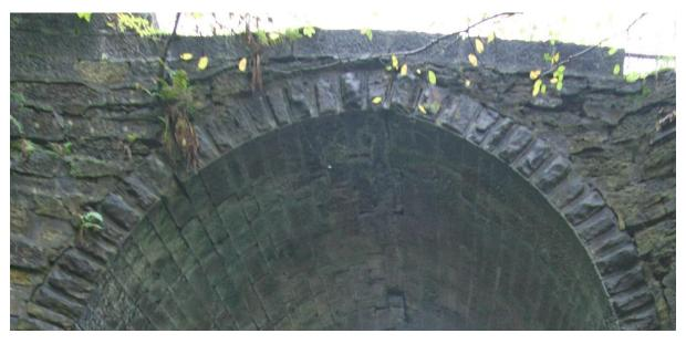
Now we can see clearly what is happening. Just to the right of the crown there are two joints wide open at the top. There are two diagonal cracks going up from the arch at the right where the wall has lifted on the arch. At the left, the stones are better bedded and the pattern is rather different.
