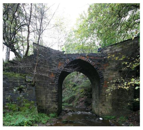
A pointed arch? Not originally, that's for sure. This is on a flood plain, but the river is right at one side against a cliff so the road comes across at high level and has to be approached on a high embankment (to the left in this picture).
