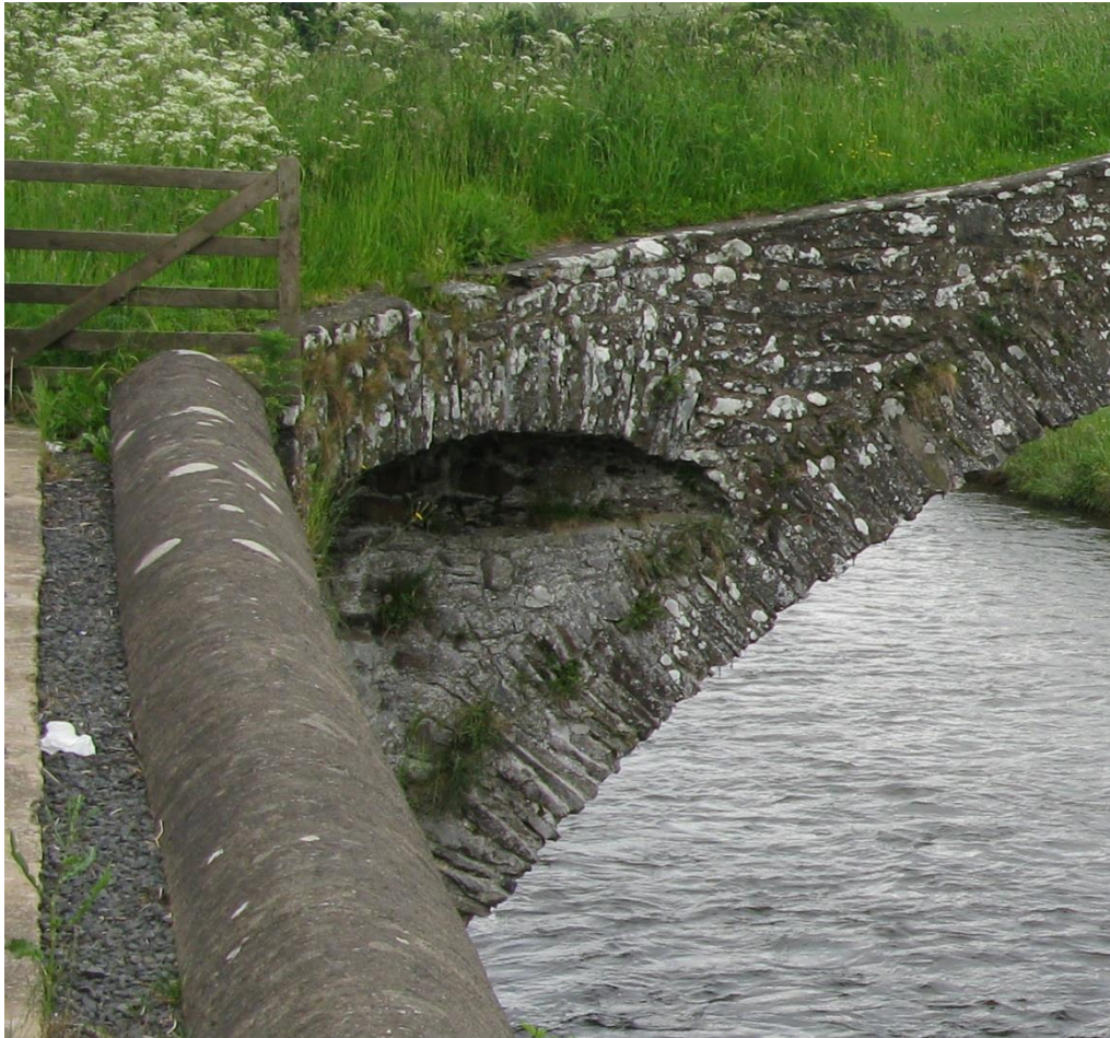
A closer view of the concrete lined arch is also worthwhile.
