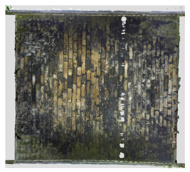
Here, the combination of moving and turning the camera resulted in limited overlap between photographs. The aim is generally for 2/3-3/4 overlap in both directions. This can be difficult to achieve at close range when working with a single camera, which is one reason that we use rigs carrying multiple cameras for our commercial modelling work.
