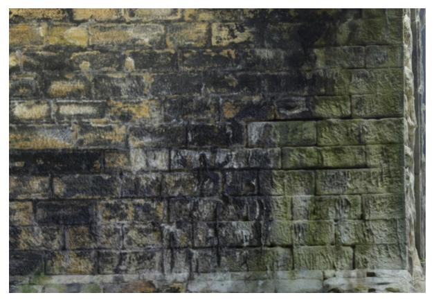
At the other end of the span there are some empty bed joints. A closer look shows stone that has been washed away from the edge of the joints. There has been a lot of water through here down the years.
