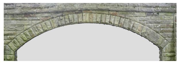
If we zoom in a little and look at just the ring, there are a number of interesting details. First, note that the voussoirs are of apparently random thickness. The joints vary in thickness too both from joint to joint and through the depth of a joint. Most of the voussoirs seem sensibly wedged but one or two near the crown look parallel-sided.
