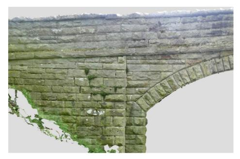
Above the abutment at the left of the main elevation, there is a further step in the parapet which just might be real but it seems unlikely. In the wing wall below there are some wide empty joints and some modest vegetation.
