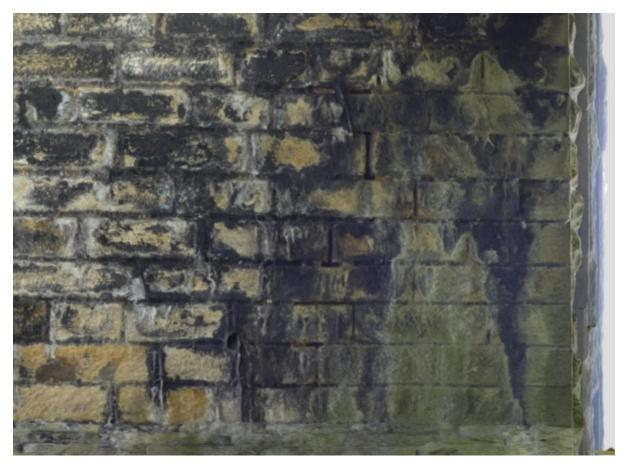
Looking closer at the soffit, the interesting features are in the corners. Here we have some completely empty perpend joints, though the bed joints are largely full.
