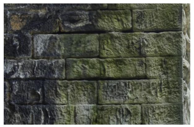
There is a further line of water run closer to the springing. I presume this is coming down the inside face of the spandrel wall to get to here.
