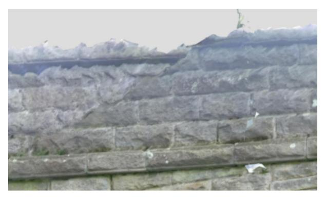
The string course is straight and the parapet has a step. The difference develops over a sloping line. This happens where there are photographs from two different directions that are only indirectly linked. Cumulative errors result in an offset between parts of the model coming from the two sets of photographs. The lower detail and quality to the left of the line suggests that this area is coming from more distant photographs.
