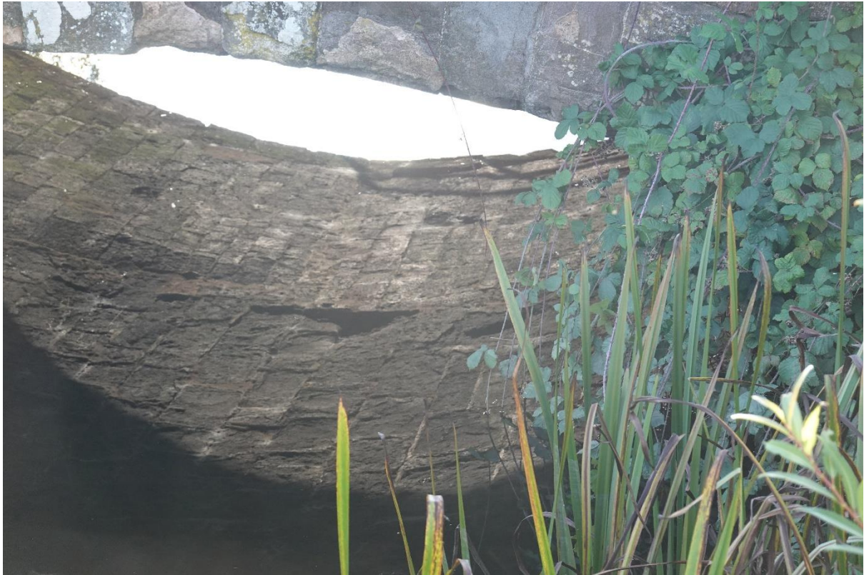
Nearer the middle of the length is another flood arch. As flat as the rest.
