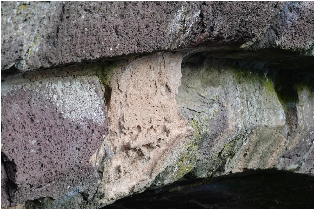
This stone has a complex story to tell. Different material, badly eroded but proud of the rest of the arch. Has it swollen or was it a later insert that was placed without care to dress it back. Perhaps the mason knew it wouldn't take kindly to the run-off from the surrounding volcanic material.
