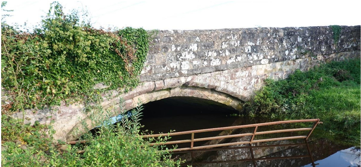
At the west end is a flood span that looks remarkably flat, but is obviously mediaeval.
