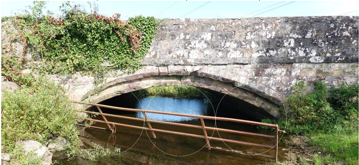
Overlaid with circles along the springing line we find a span rise ratio of 6. Really unusual.
