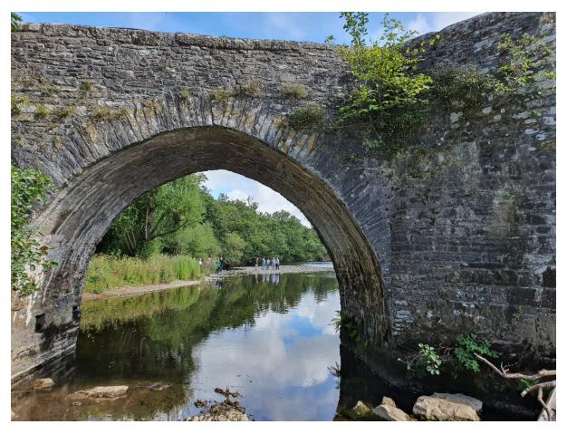
Looking square through we can see that the arch is made from selected but not tapered stones. The builders have nearly managed to follow the curve but left a broad wedge to fill at the, slightly pointed, crown.
