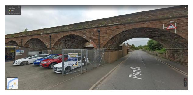
There are several things to note in this image. There are four modestly skew spans of 40ft (12.2m) span and 10ft rise. I would expect that span to be on the skew (parallel to the arch edges, not "square" to the pier faces), the same centres surely having been used for both viaducts. I hadn't thought that far when I was there 20 years ago.
