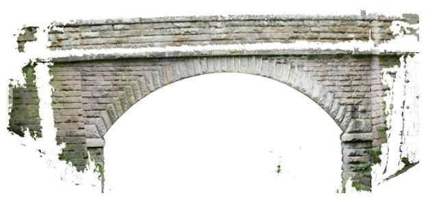
This orthographic elevation suggests that the arch is circular on the square, despite the very high skew. A square view of the spandrel wall looks rather flatter, with the curve increasing slightly towards the springing. Among other things, notice here how the voussoirs are lozenged shaped. This is what you get when you cut through a spiral on the skew.
