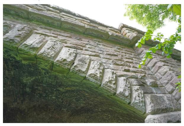
At the corner above, the skewback naturally forms a solid piece for the arch helix to sit on. At the opposite corner, construction is much more complex, with a double voussoir cut into the single stone.
