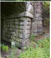
Skew bridges, road over rail, are usually built on standard square span centres except when the skew gets so severe that setting it up becomes expensive and complex. If the standard bridges are segmental (as here) square centres will result in a stretched, elliptical skew span. I suspect that this view is showing a squashed ellipse on the square which means circular on the skew.
