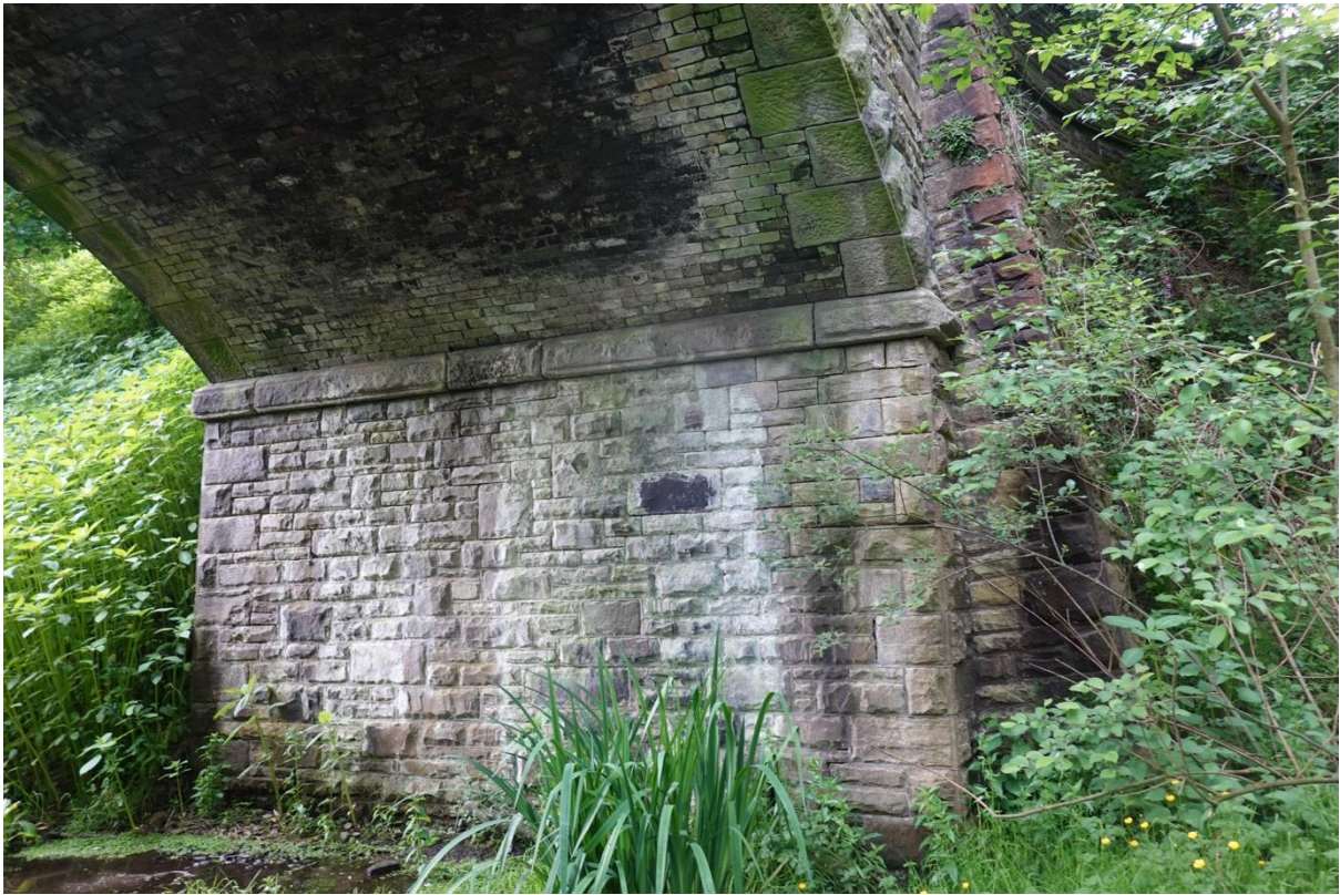
The black smoke on the sheltered soffit has been washed off near the arch edges, presumably because of water penetration from above.
