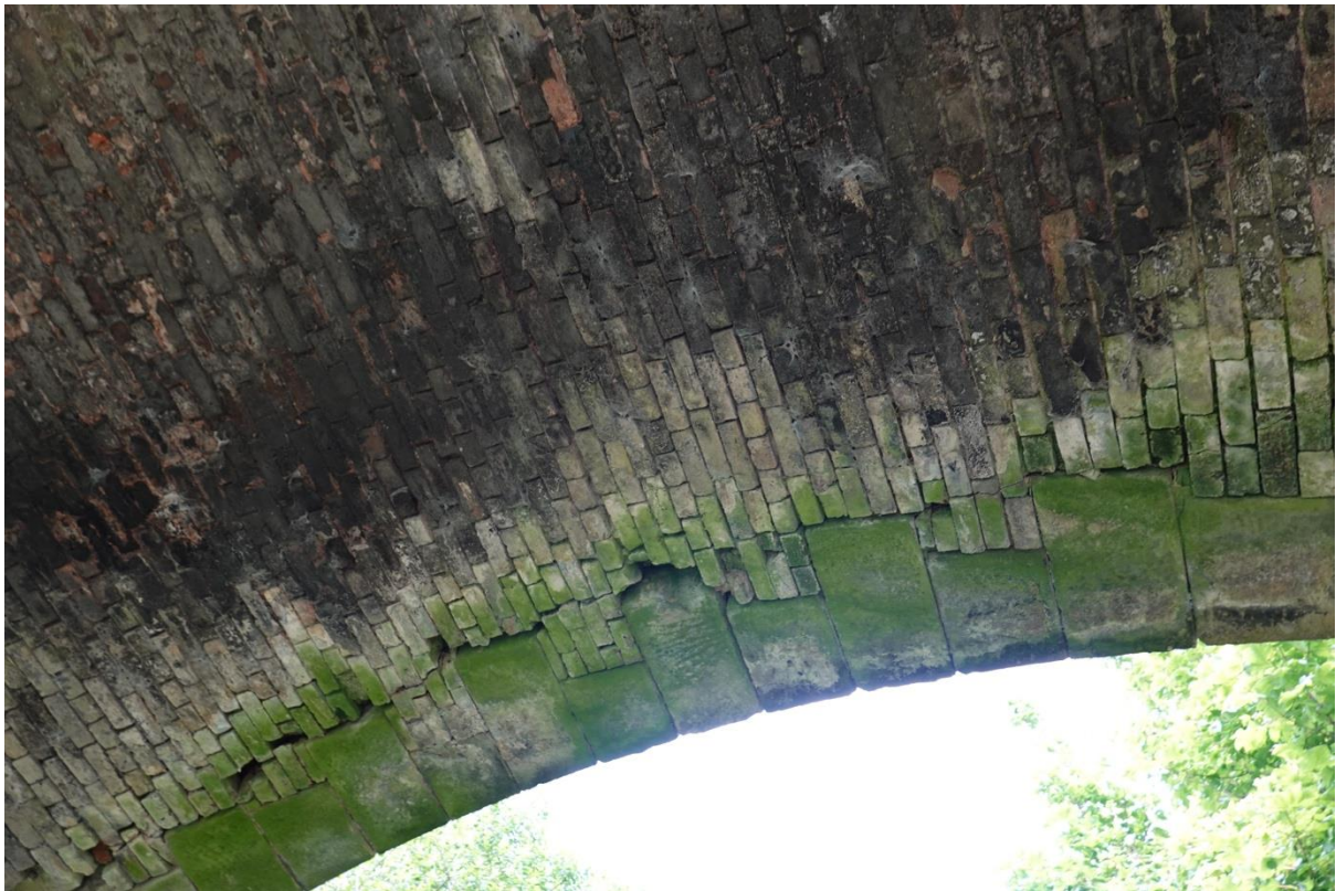
The black smoke on the sheltered soffit has been washed off near the arch edges, presumably because of water penetration from above.
