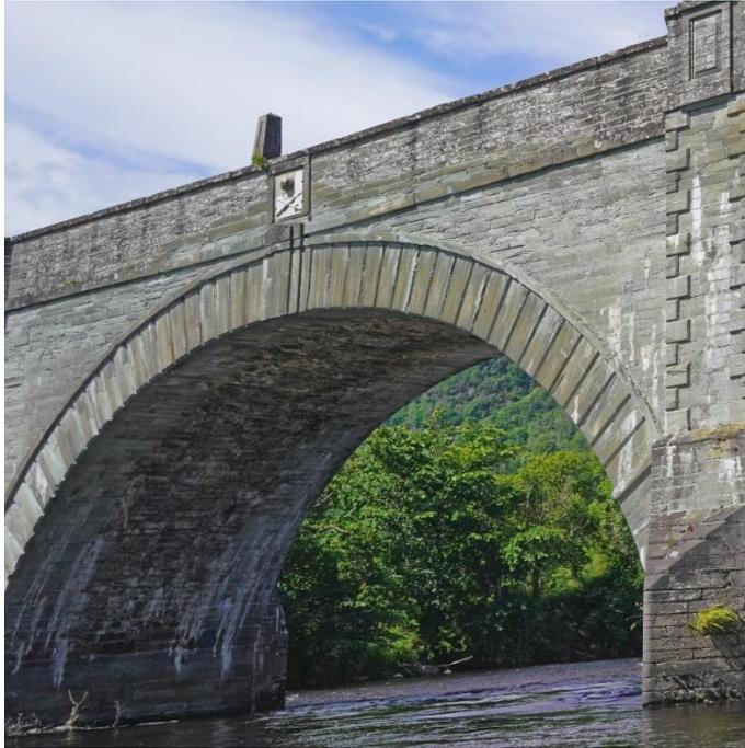
The wet patch is just about visible here at the  $\frac{1}{4}$  span point. In one recent flood, the water reached this level. That will have sought out any weak mortar and removed it. Perhaps it was weakened by those heavy vehicles nearly forty years ago and the damage is only just showing. I certainly cannot imagine why the damage should be at diagonally opposite points in the span.
