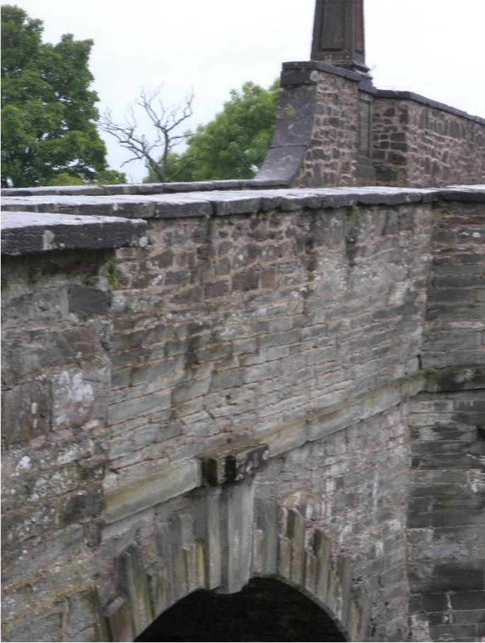
The string course in the foreground original also formed a kerb on the inside and marks the original road level. The present level is roughly where the parapet changes colour. A look over the crown from mid span provides an alternative view.
