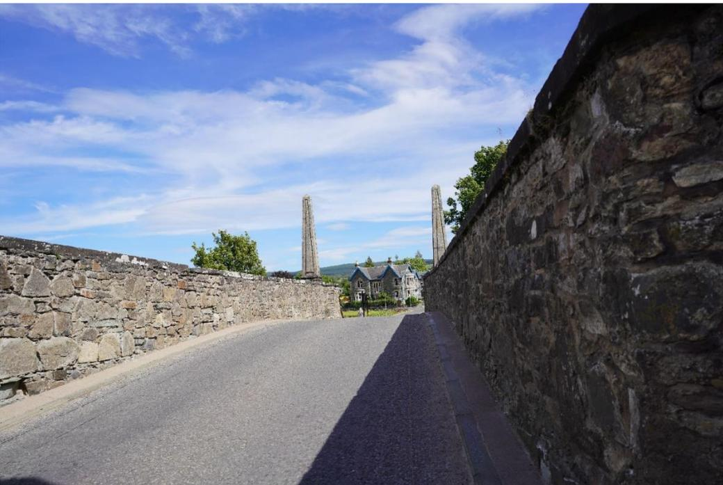
The dip in the string course is more pronounced than in the parapet top. The drop of the arch when the centres were removed was non-trivial. The parapets were not completed for nearly a year, so the sag there represents longer term movement.
