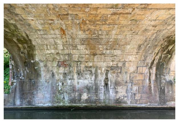
This image shows the tightly coursed stonework in the arch. The quality of the stone is clear from the tooling marks still sharp after 200 years of weathering.
