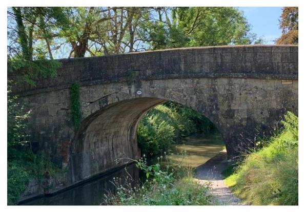
The bridge is of ashlar throughout. The arch is three centred to provide headroom, at one side for the horses and at the other for the barges.
