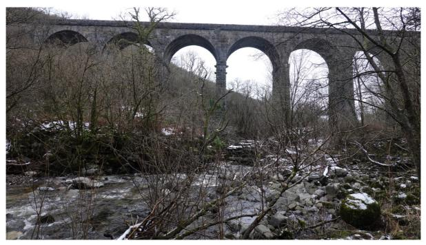
The piers of the river span are founded directly on exposed rock. The west bank pier (right photo) straddles the edge of the shallow gorge where the river does a dog leg. I didn't get a view from downriver. I wonder how much of the undercut on the east bank (left) has developed since the viaduct was built. Presumably the other piers are also founded on rock.
