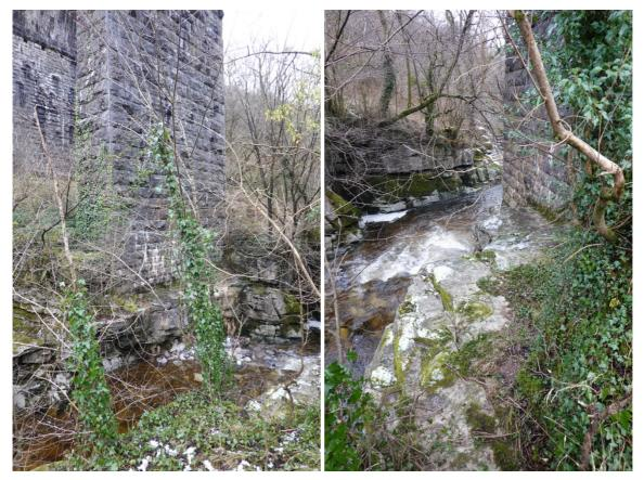
The bridge is built of local stone, reportedly direct from adjacent cutting, perhaps to the east, where the track bed runs along a ledge cut into the hillside. That stone is not the most robust; a scattering of small shards is found on the ground around the piers.
