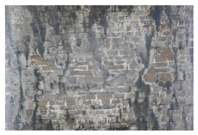
increase in flow through the joints to the upper and lower edges of the frame. The drains seem to have been placed rather high relative to where the main flow starts.
