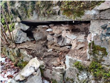
A close look gives a nice view of typical wall construction, with two faces and a core of shards, mortar, and considerable empty space. No match for the relentless power of unchecked tree root growth. A look past the end of the parapet highlights the scale of the valley.
