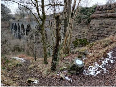
A slightly zoomed view nicely captures the over line bridge to the west, and shows the slope, not previously so obvious. The stone courses are independent over each pier, and meet in a jumble over the crowns. Note again how low over the pier the drain hoppers sit.
