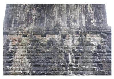
There are remarkable lime growths on the upper part of the pier in some spans. I thought these might be nests until I was able to inspect the photographs. The pier faces are battered, and the stone rusticated. The drips must have landed where the stone protruded furthest to begin with, and the lime built from there.
