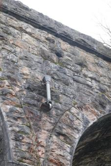
Drainage is provided over the abutment, not universal, but probably wise given the scale of the abutment here. Another curiosity in this view: there are no putlog holes at the abutment.
