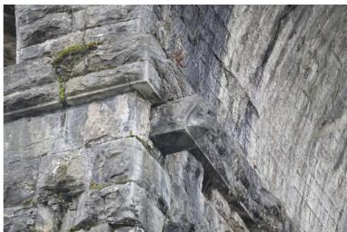
The arch rings are in less than perfect condition. Not terrible, but lots of water flow and clear lines of weakness stepping along perpend joints.
