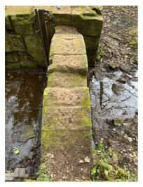
intrados. I think the difference may be nearly 100mm. Could that low stone lift the arch enough to cancel that out? I suspect not but I ... must ... resist ... getting further into the geometry of this right now.
