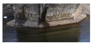
The concrete skirt at the base of the pier isn't level. How did that come about? It rather looks as if the base of the concrete might be visible with clear space between here and the current river bed.
