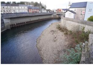
Note the silt and gravel (and general detritus) under the smaller span. If we look upriver, we can see the reason for that. We have expensive looking hard engineering works, holding the course of a river that wants to move. It can't get past the sheet piles, but it can still dig down on that side and dump material on the inside of the bend.
