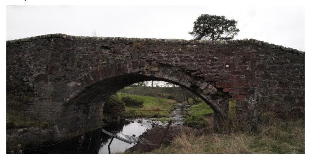
Notice also that the left abutment and lower wing wall is concrete. The flow is still hard on that side, so presumably there was severe scour damage here in the past.
