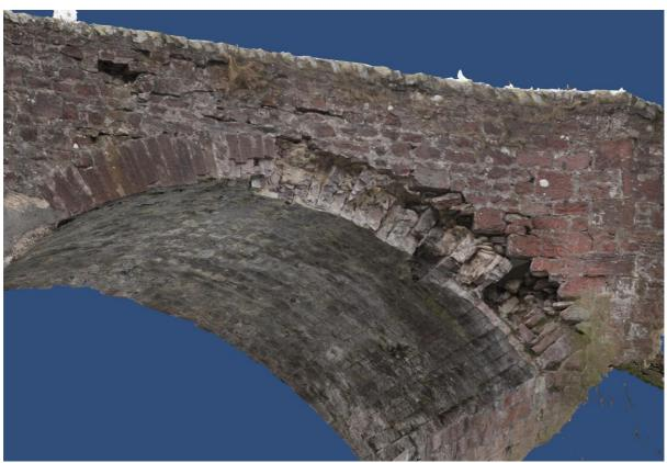
Above the right quarter point in the photo above, where the edge of the ring has gone, part of the inside face of the parapet has fallen off too. Possibly related, possibly not. Notice the rubble inside.
