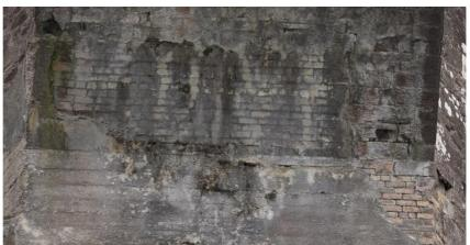
The damage to the upriver side follows a diagonal line from the abutment to the crown and then up through the spandrel wall and parapet.
