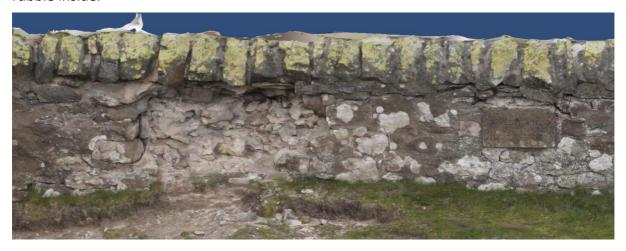
And speaking of rubble, the ring damage gives us a glimpse of the backing. The stones of the ring are broken up, and it isn't clear that they were all originally through stones. But in the nook above the ring and behind the spandrel/wingwall the unshaped rubble backing is visible.
