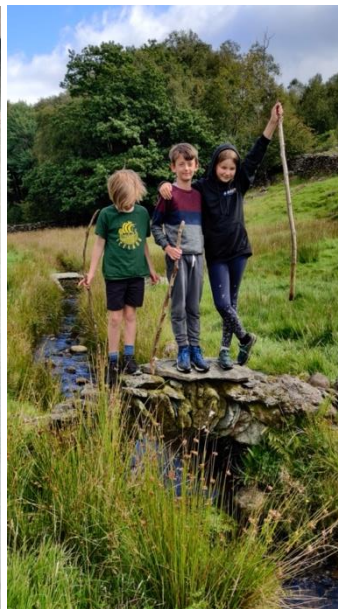
Dry stone bridge. People often ask about the hump-back bridge over the Black Sike at the foot of the fell. It was built by David Lascelles and James Hesketh-Prichard in 1992 as part of a scientific exercise to create a “dry” self-supporting stone arch. It has survived because, as an architect friend told us, “the stones cannot fall because they have nowhere to go.”
