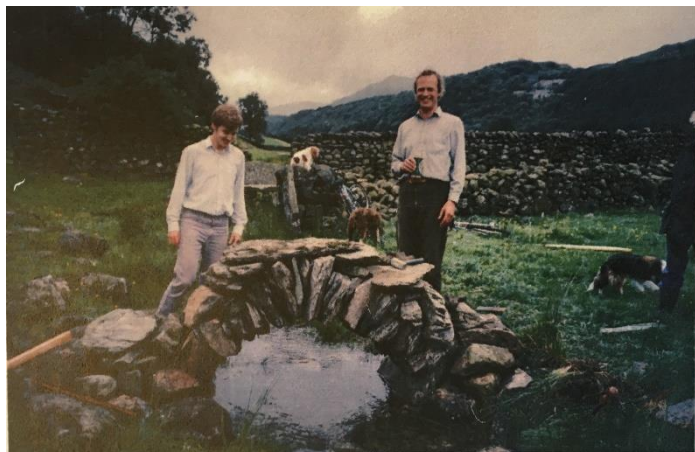
Dry stone bridge. People often ask about the hump-back bridge over the Black Sike at the foot of the fell. It was built by David Lascelles and James Hesketh-Prichard in 1992 as part of a scientific exercise to create a “dry” self-supporting stone arch. It has survived because, as an architect friend told us, “the stones cannot fall because they have nowhere to go.”
