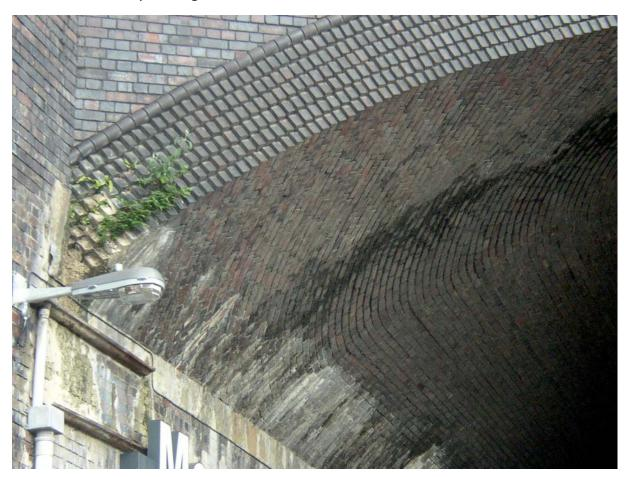
The picture above shows the nature of the arch construction. The skew angle on this face (zoom in on the map to see) is about 40 degrees. At the other face there is a much smaller skew in the other direction. The skew edges are accomplished by sweeping the brickwork round a curve so it runs parallel to the abutment over most of the width but still meets the skew edge more or less at right angles.
