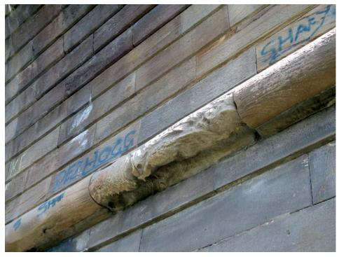
One last picture to show how the weathered stone stands alone in the structure. Clearly a function of the stone rather than the environment.
