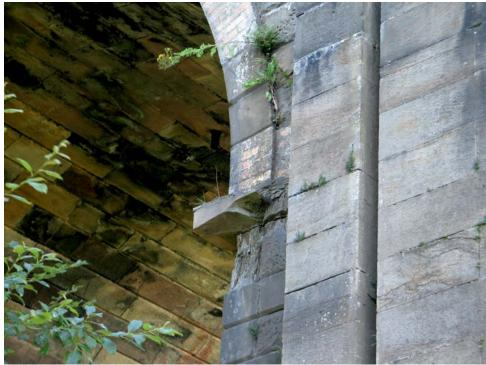
Here we see a drain at the arch crown, which is a strange idea if you do not realise that the deck is a notionally flat slab which will necessarily drop at mid span after decentring. There is a very wet stripe below the drain which might be splash from the drain itself or might be showing the line of the central void.
