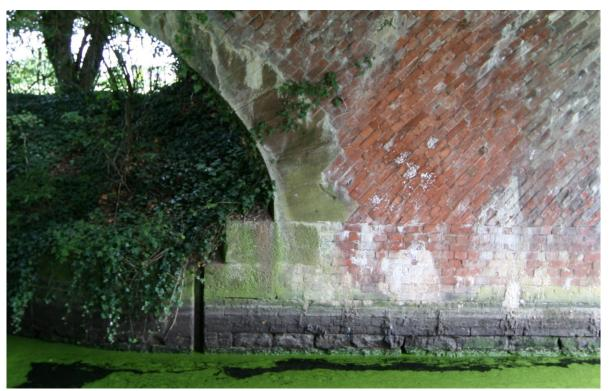
At the obtuse corner, the voussoirs are less determinedly brought into line with the helical coursing of the bricks.
