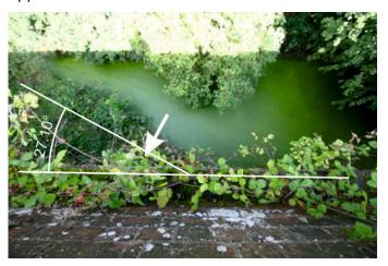
Here I have highlighted the line of the bridge and of the canal wall The latter is less obvious so there is an arrow to point it out. In this sketch view the angle is measured as 27.1degrees so the skew angle is truly 63 degrees.
