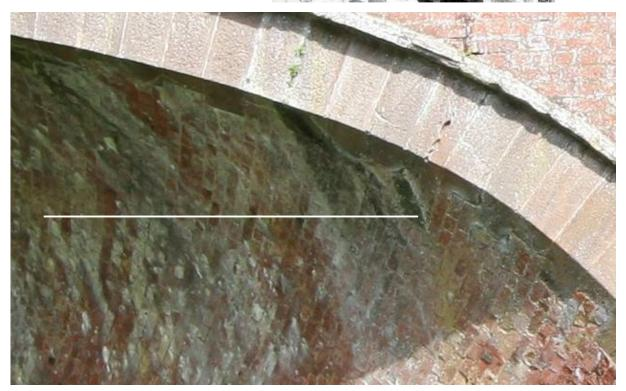
And just a final shocker, here is a photo taken from the sharp edge of the abutment! If you look closely, you will see that the nearer part of the arch has a different shape from the far end profile. This is the reverse view of the profile changes noted on page 1
