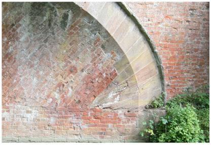
The edges have stone voussoirs keyed in to the main brick ring. The voussoir angles are very complex, especially in this corner where it is necessary to get from horizontal to the main spiral. In the spandrel elevation it is possible to see the lozenging of the exposed face of the voussoirs caused by cutting off a helical face at an acute angle.
