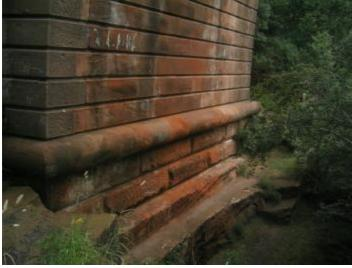
The scale of the stonework is seen from this closeup of the abutment.These Voussoirs are about 0.5m thickand some are nearly 2m square. Lifting them the 60m from the river withthe hand winch on the Gantry crane must have been a serious undertaking.
