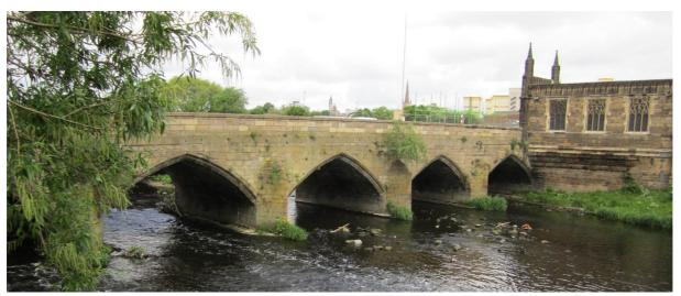
Here are 4 spans of the 9 spans. There is another hidden behind the tree and four north of the chantry chapel which actually partly blocks one span. These five arches have flat soffits whereas the four northern ones have ribs (see below). This surely indicates an element of reconstruction of even the earliest parts.
