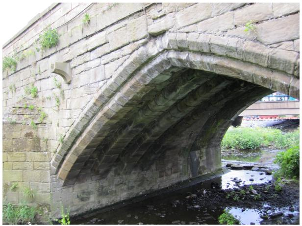
The ribs seen here are chamfered on the outer edge but square in the middle. If the ribs and gaps are equal (as they appear) the width of each will be 18in (450mm) with a 9in edge (225mm) corbel chamfered by 6in(150mm). The other dimensions then suggest that both the ribs and the arch are 9in thick.
