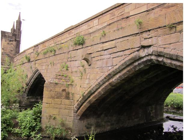
Here, there are obvious signs of earlier distress, and also of previous basic configurations. The original stonework is coursed making use of different bed thicknesses in the quarry and carrying each bed through the whole bridge. This was typical of the imported cathedral kits that were brought over from Caen. Tracing the courses through this picture we can see:
