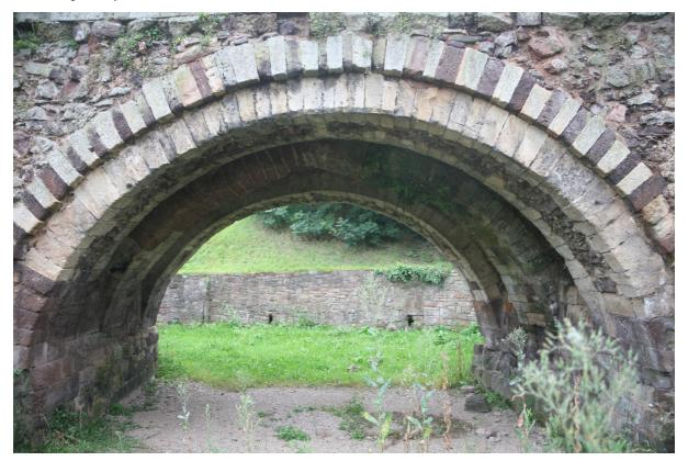
The ends of the arches are vertical, or nearly so, and required no support. They could therefore be built in rubble. The photograph below shows that the lowest portions were of dressed stone. This was probably to maximise resistance to the damaging effects of flowing water. Above this dressed stone is a layer of rubble masonry and above that, much larger stones were used.
