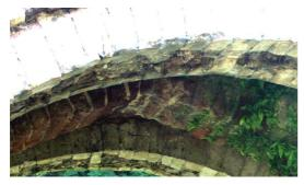
A closer look at this central section shows that it has probably been replaced and the masons had trouble fitting the rib properly. Perhaps they were working in haste to restore a badly needed road.
