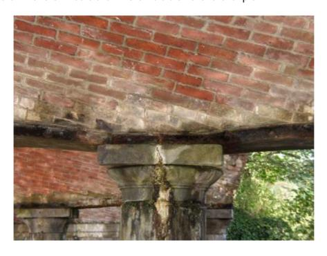
But none of that is the reason for showing this bridge. The important thing is what it has to teach us about skew arch behaviour. The established view is that skew bridges try to span square. Even if that is true, the centre of thrust at mid span must be at the centre of the bridge width. Drawing that effect shows that the resulting forces on the piers create a substantial moment in plan (below).
