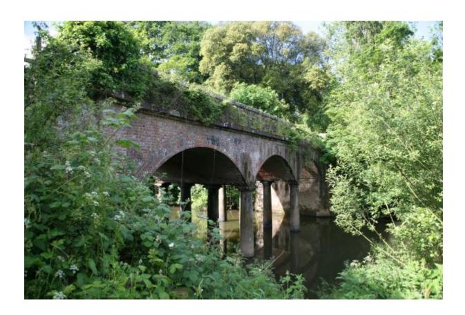
In this shot you can see that the bridge is skewed but the more important issue is the piers. Each pier is four columns of granite. Above that are cast iron shoes providing a base on which to build the arch skewbacks.
