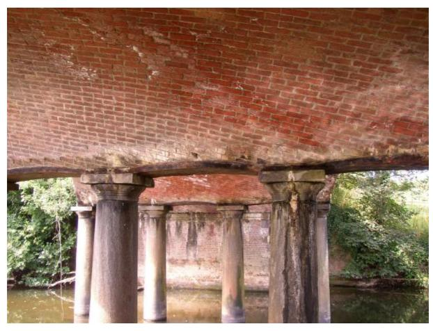
You can see, here, how the shoes divide in the middle of the piers. Any joints in the stone are well disguised. Indeed, it was only on closer examination of these photographs that I detected the illusion created by marking up brick shapes on the stone face. A closer look, below, shows how the cap stone of the pier column has split. It also shows the change from real to drawn bricks. That is even more visible on the further pier.
