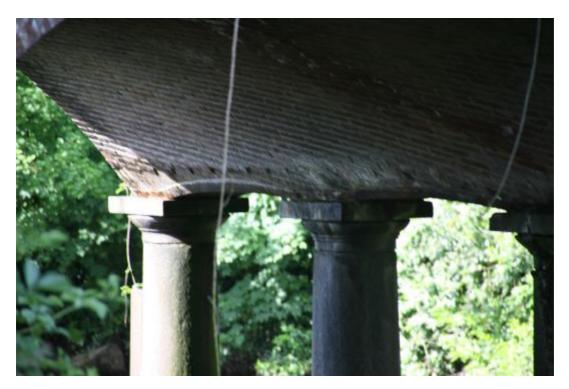
The join between the stone skewback and brick arch is very visible here.
