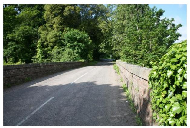
These are some of the flattest parapets I have seen. A sign of a very robust bridge. The stone copings finish it well. I have never before seen a parapet with a stepped inside face. I think the lower step, just above the pavement, is the inside edge of a stone string course which appears on the outside.
