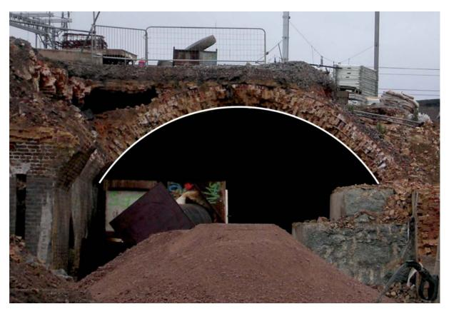
Here I have fitted a 4:1 circular curve. Perhaps it would be useful to present the calculation.
