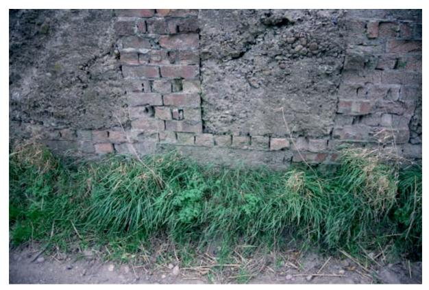
A close up of the cut face shows relatively low quality concrete and even the brickwork has mostly empty perpends.
