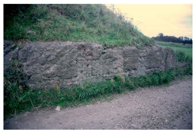
The other abutment has been cut off revealing the internal construction.
