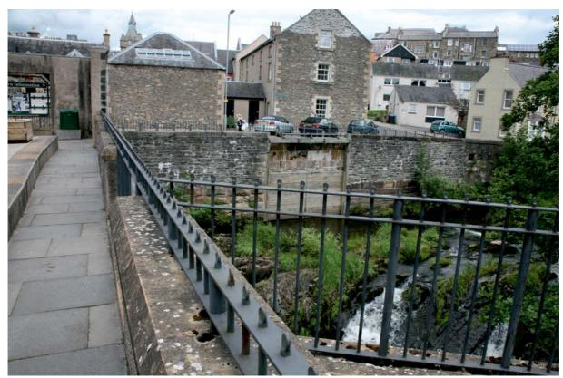
To the left here you can see that there is a worthwhile waterfall in front of the arch as well as the drop beneath it. It seems that the mill was powered entirely by the local drop without the benefit of a weir and leat. The water is taken off just above this fall through the blocked sluice shown here. It emerged (presumably) from the partly collapsed tail race tunnel below.
