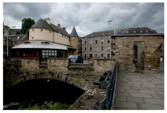
The upstream face is square. The extent of the structure is somewhat disguised by the very wide angle shot (14mm on a Canon EOOS5D) but the rocky bed is evident as is the extent of the drop in water level over this short distance.
