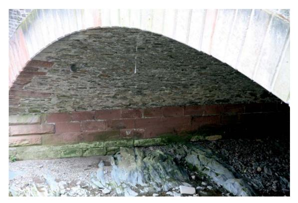
The skew is modest, but quite visible in this shot. The dressed stones are only in the face and the abutment walls. The arch proper is built from random stone straight from the quarry with correspondingly large mortar joints.
