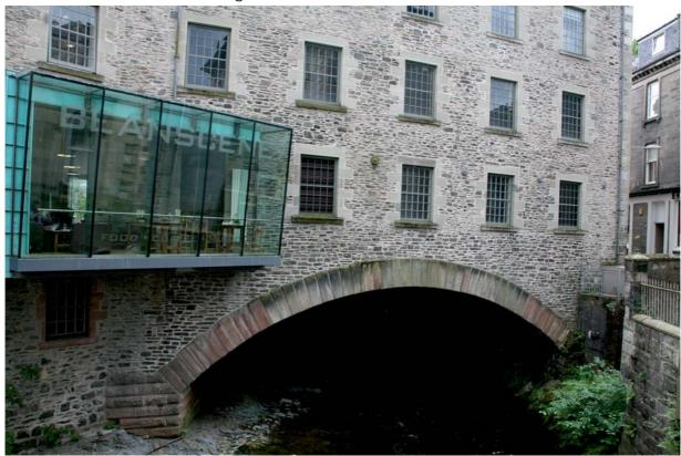
Rock is exposed in the river bed so foundations were clearly not a problem. These skewed face has nicely dressed voussoirs of uneven thickness, with some thinner voussoirs near the springing.
