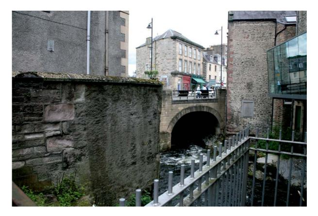
The bridge downstream has its own interest. It is not easy to photograph but this shot shows the arch to have a varying radius without reaching the vertical at the springing. this view is severely foreshortened and yet the centre of the span still looks quite flat.
