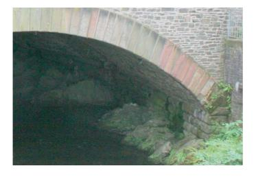
Cropping this picture and pushing the light severely reveals a kink a few metres upstream of the arch face. The remainder of the structure is essentially square. This skew arch constructed from random rubble surely gives the lie to the idea that bedding of the stone or brick is structurally significant in skew bridges.
