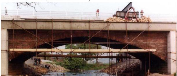
The bridge is recorded as having a span of 18.299m, rise of 2.845m and a ring of 0.711m Silly sounding numbers until they are re-interpretted as 60ft, 10ft and 28in. Of course, the arch sagged when the centring was struck so the rise measures 9ft 4in! The road surface was essentially flat and the cover a mere 200mm at the crown.
