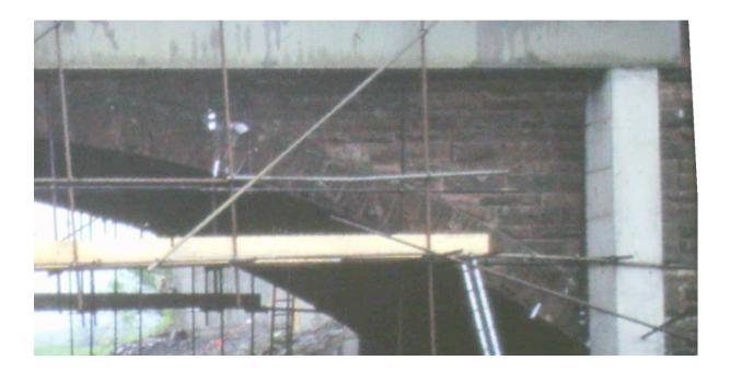
This is part of the first image, cropped to show detail. The overlayed white lines show the slope of the beds where the arch has sagged during construction of the spandrel walls.
