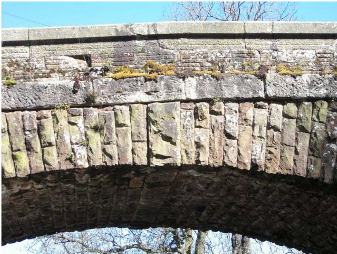
This looks like an expressed keystone, but it is surely not in the centre of the span. The top edge has a distinct slope. Looking back at the first picture leaves me wondering whether this is a mason's joke!
