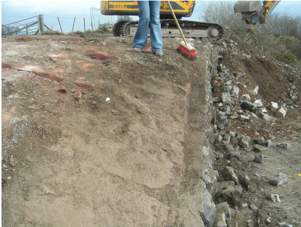
This very small shoulder supports the surface skin of the spandrels. Behind that dressed stone is a random rubble wall.
