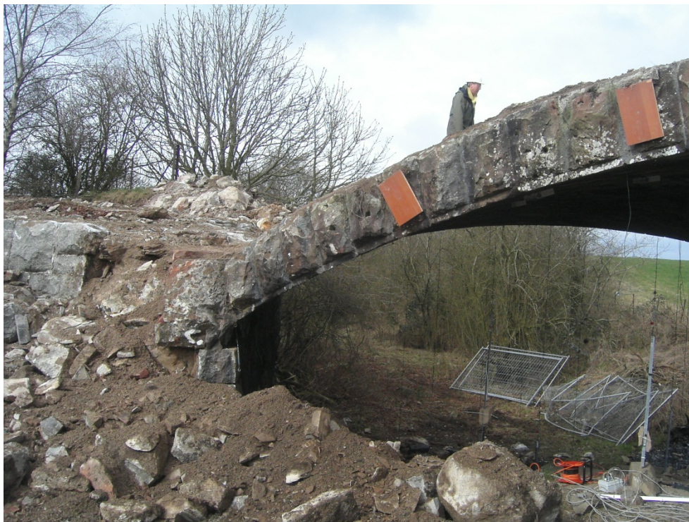
The very shallow depth of the arch itself is made abundantly clear by this edge view.
