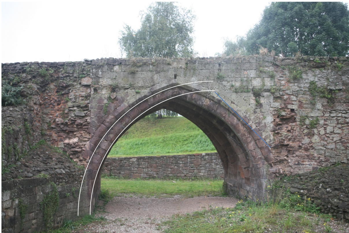
Figure 2 Exe bridge pointed span with circular curves
