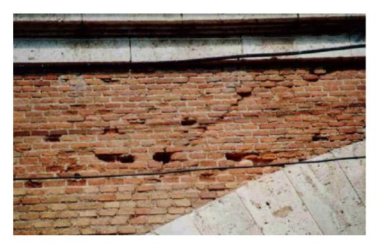
This, yet closer look is obviously a different span. The line at which the weathering starts is very clear. There appears to be a diagonal crack in the brickwork but it might just be a construction joint, perhaps where the skilled bricklayers worked away from the ring and produced and easy edge for the improvers to work from.
