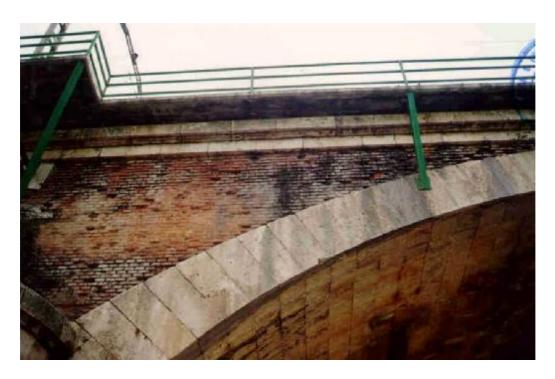
A closer look shows more of the nature of the weathering of the brick. It also shows clearly that the expressed ring (at least) is tapered, beautifully fitted and has tight joints.
