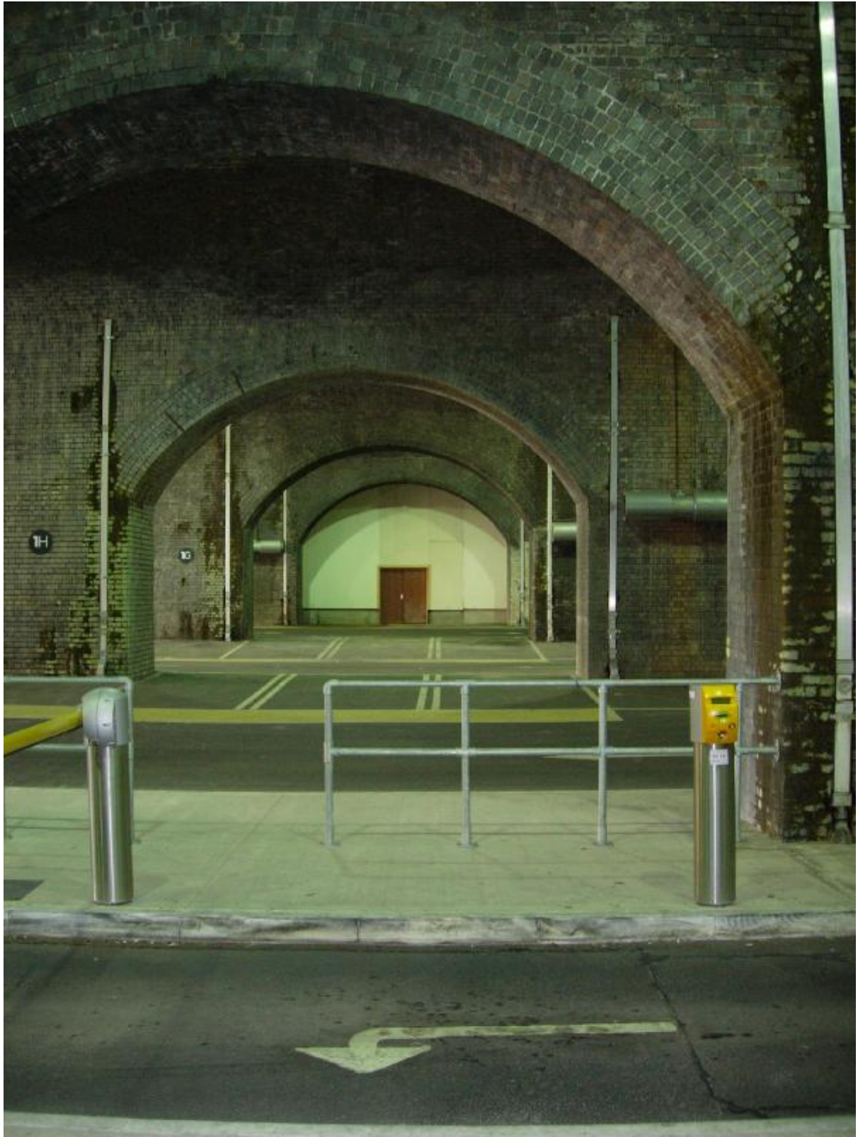
The goods sidings ran this way, parallel to the tracks above. There was a traveller at the end and a wagon hoist in the corner.
