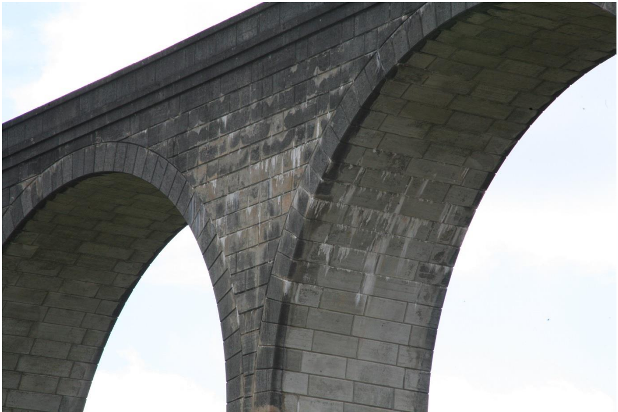
In the closer picture, note how the lime runs match on the soffit and the spandrel. The arches were almost certainly filled with concrete to this level.
