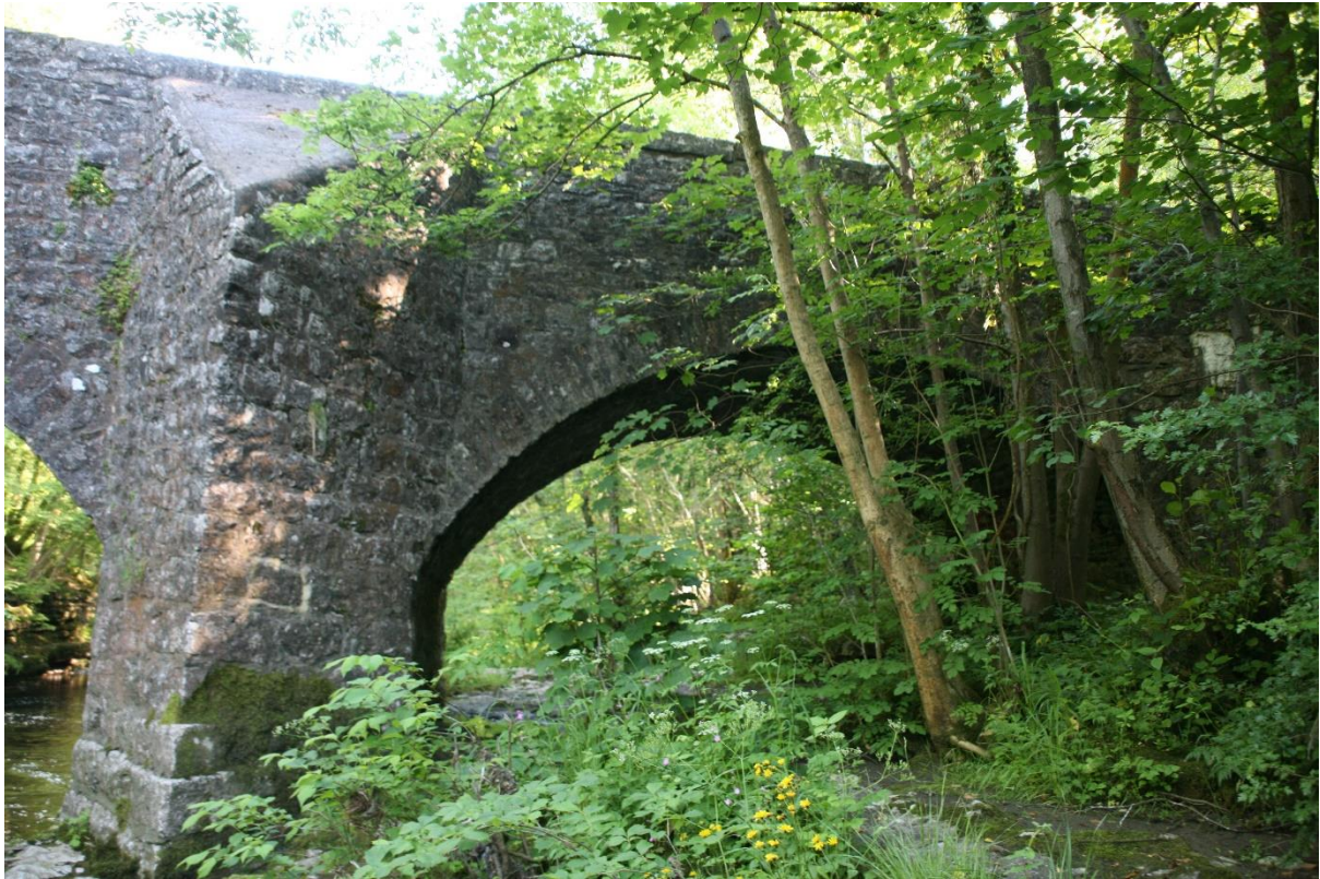
This side span was built in a single width.
