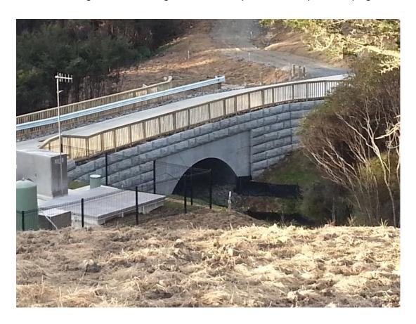
And to give an impression of speed, the arches were installed one day and this concrete saddle the next followed by fill the next day.
