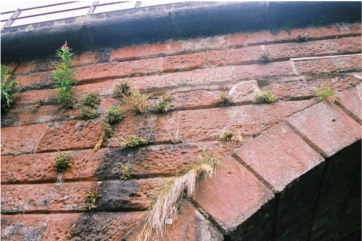
At Crawick viaduct, the voussoirs feature a series of parallel chisel marks creating longitudinal lines. The spandrel is moderately rusticated but V jointed.
