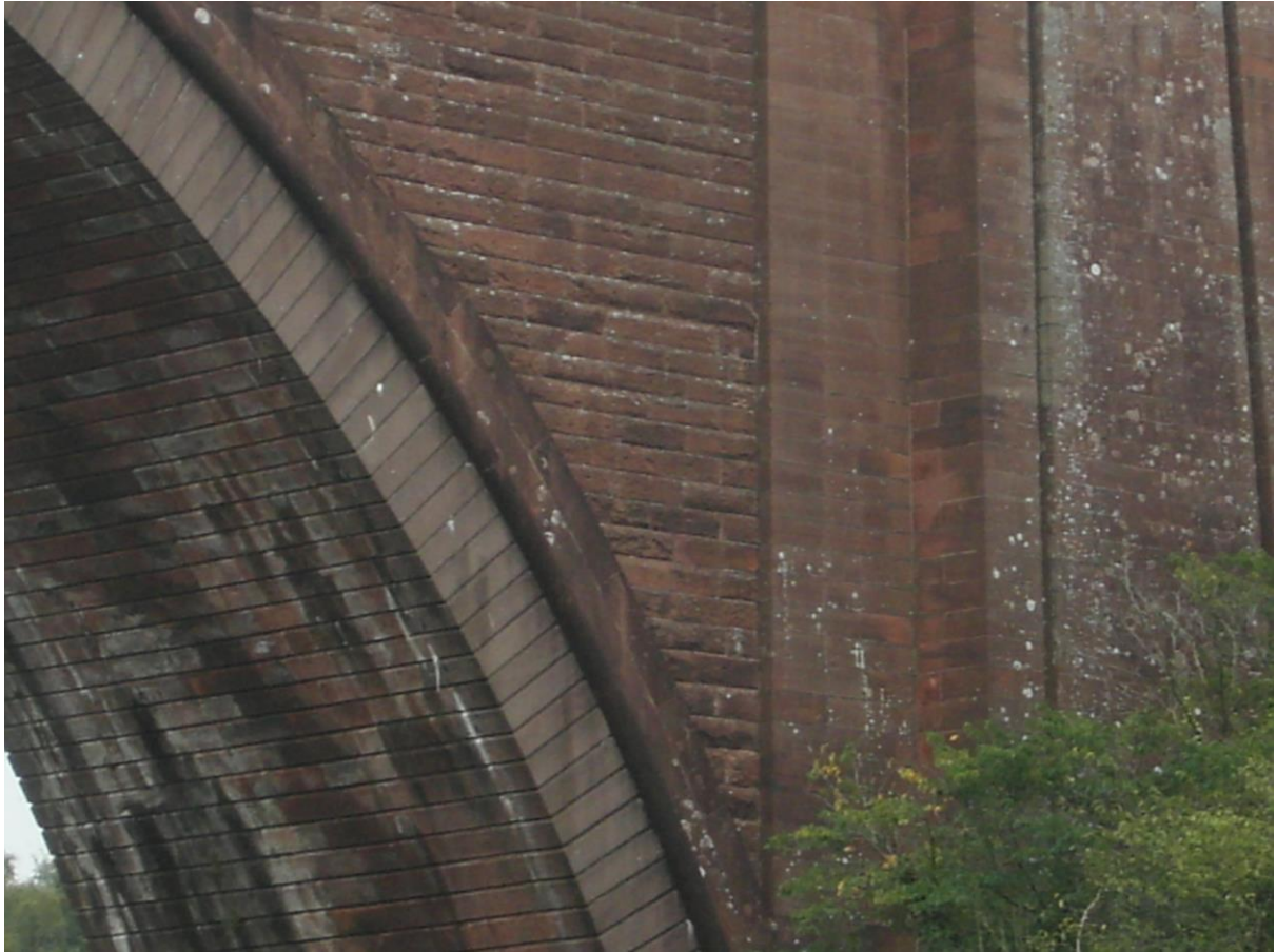
At Crawick viaduct, the voussoirs feature a series of parallel chisel marks creating longitudinal lines. The spandrel is moderately rusticated but V jointed.
