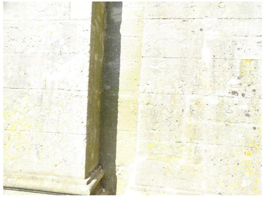
Otherwise, the stone is in remarkably good condition, with the mason's marks still clearly visible.
