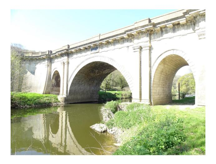
There are many indications of the hand of John Rennie here, for example, the pilasters and the scale of the corbel.
