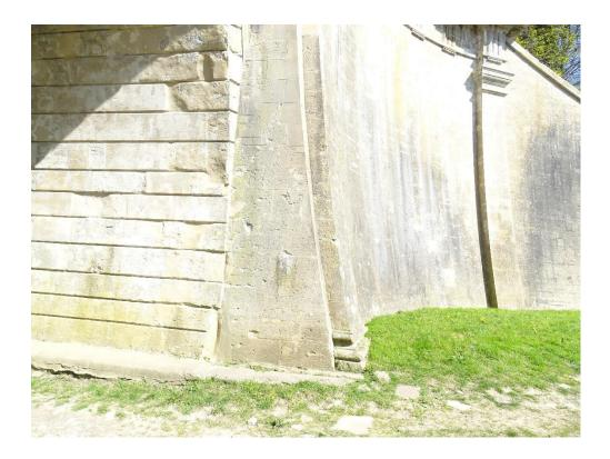
The sweep on the wing wall is very elegant as well as structurally welcome. The masons must have been a bit tested by ashlar in a double curved surface like that.
