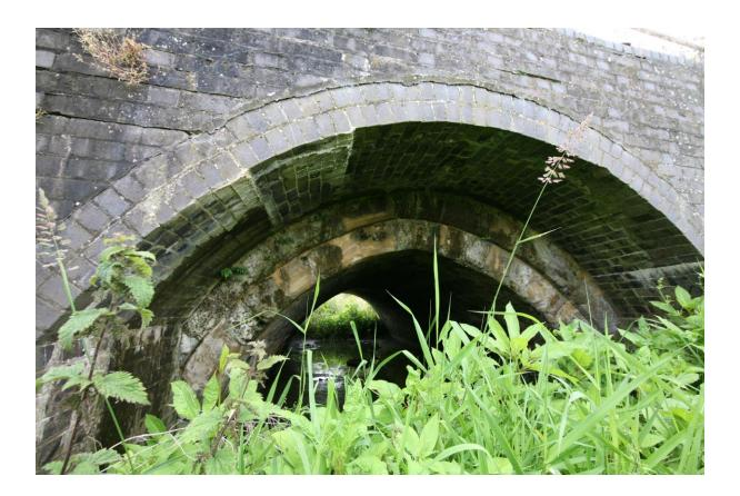
Here on the west side, standing on the very wide extension we can see that the old arch has also been widened but on this side they get wider to the north. The band of stone immediately below the copes on here must be different. Tremendous growth of lichen.
