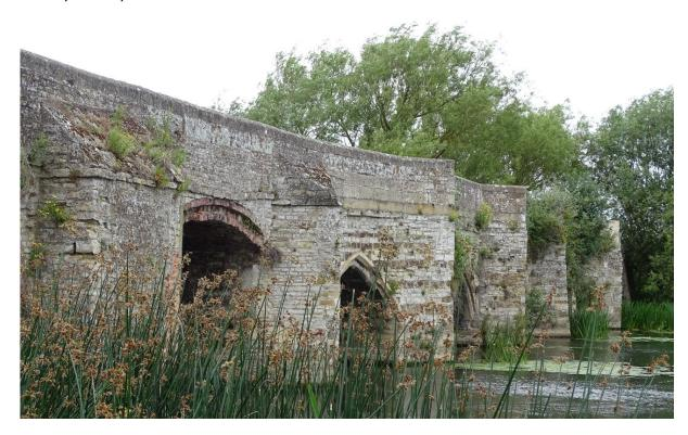
To the south of the high span, the ribbed arches return but have further brick arches in front of them.
