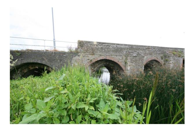
The brick extension in the flood relief zone is wider yet, and here we can see through to a substantial widening on the other side.
