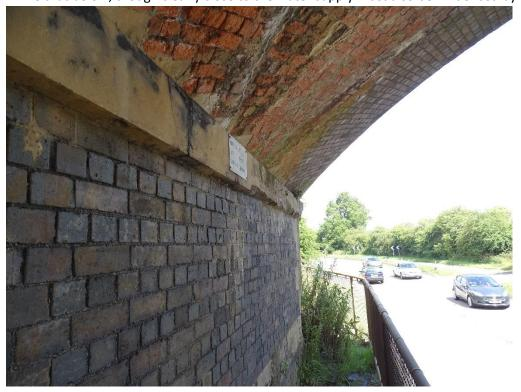
That becomes clearer looking from the other side where there is a fracture running from the edge of the abutment to the springing intrados.
