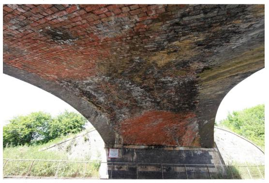
This shot is taken from close to the bridge centre line and shows almost the full width. Cracks are visible (some actually marked with chalk) that look as though they run parallel to the tracks and possibly directly under the rails above. It is also from the Sony, zoomed in a little, perhaps to about 35mm equivalent.
