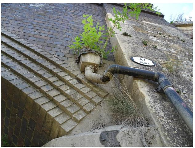
They are positioned fairly low, so almost certainly the drain slopes uphill into the structure. Here we see a considerable flow of mud which has blocked the drain. There is now a tree growing.
