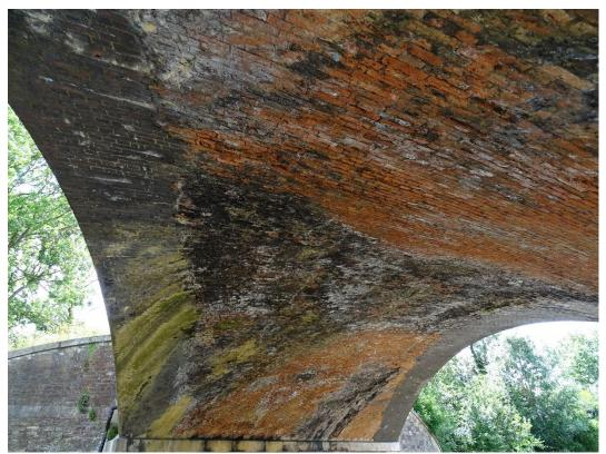
A look at the soffit shows that one edge has been completely rebuilt. Note that these photos are taken with a moderately wide angle lens, 24mm (equivalent, actually rather shorter in reality) on a Sony HX400V, so they distort the image slightly but show almost the whole soffit in enough detail for a close examination. Putting alongside that what can be achieved with a 14mm lens on a Canon EOS5DMk2 is perhaps worthwhile.
