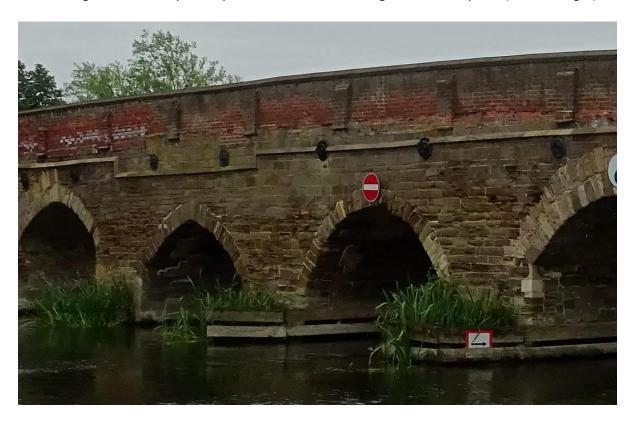
Looking more closely, these two spans both have single rings and are set very low. The right hand one is slightly higher and has a very irregular shape so perhaps it, too, is a replacement. Note how much higher the adjacent spans spring.
