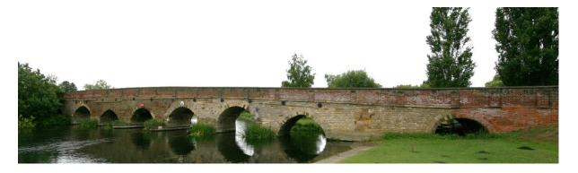
This view from downstream shows only a few of the arches. Even here, though, the multiple patching is evident. It seems likely that the low span second from the left is more or less original. The lower string course actually corresponds with a shadow string course over span 2 (from the right).
