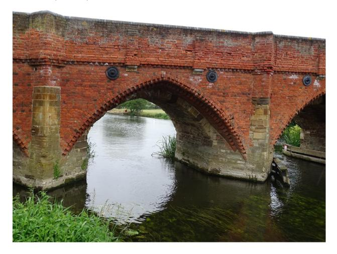
So the widened section sits entirely on the old cutwaters. Here is something I had never thought of before. The further out on the cutwater, the bigger the span. The strass levels are therefore going to be bigger on the outside edge and no matter how low the stresses are, creep is likely and the widened section will slowly lean out from the rest. The height of the main arch springing above the water is also obvious here.
