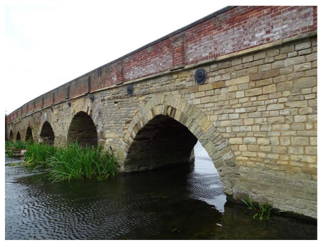
This near span, though double ringed is set very low and pointed. The two rings spring from different levels and I am tempted to think this has actually been under-ringed rather than rebuilt. Looking at that dark band close over the arch, it could be an old string course that has just been snapped off.
