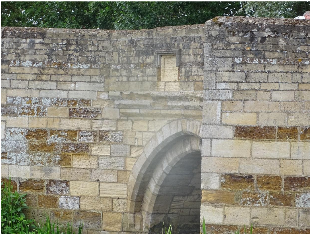
In the next span. The corbel is much bigger.
