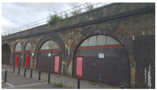
This, less distorted shot allows some of the history to be extracted. The stone voussoirs at the crown and quarter point of span 26 are apparently 18in (457mm) thick. Where it has been patched it is just 4 bricks. At the springing the pier face seems to align with the bottom of the fifth ring with an additional 3 added later. I suspect this shows two phases. A single under-ring and re-skin followed by 3 more when that didn't stop the movement, for movement there certainly was.
