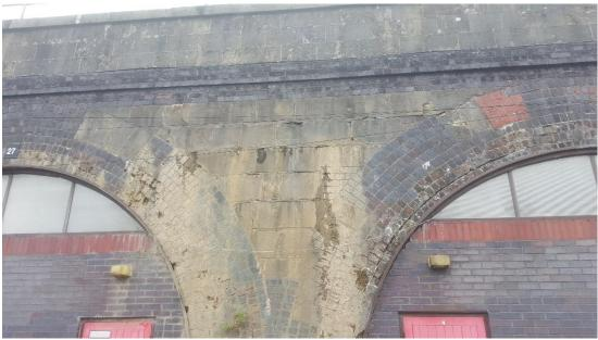
A closer look shows all sorts of things. Perhaps the most obvious is the stream of mud apparently coming from the full width, including through the ring at the stone voussoir on the left. At the next course up the stone is spalled over some length and at the right, the damage progresses into the ring. Also at the right, the inner ring seems to be separating. In span 27, the separation at the crown above ring 2 has created a path for the muddy water again.
