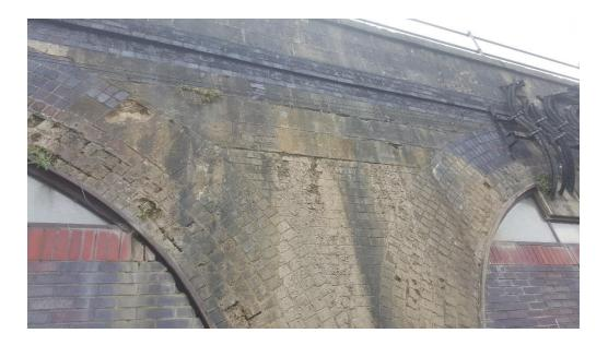
Looking to the right, the damage continues and is perhaps worse. The stains on the ring in span 29 (to the right) show that it is articulating enough to allow mud through 5 rings.
