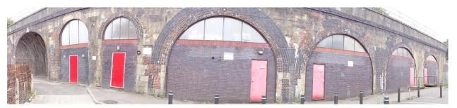
The river is to the right here. The span just visible to the left is skew and the next two short spans are closed at the inside because they are making space in an otherwise massive abutment.
