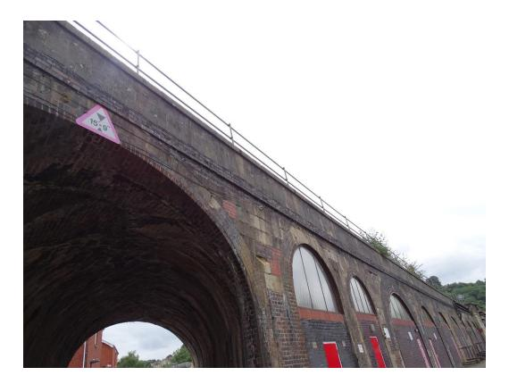
Looking along this run from the East we can see why this span has not been lined. To do so would be to severely restrict the access for traffic through this skew span. At the far end we can also see the main river spans.
