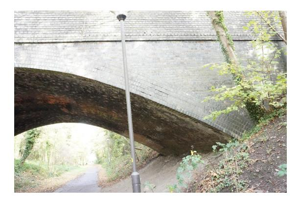
Look closer again and it becomes clear that there is substantial separation of the inner rings. But you can also see that those are metric bricks below the crack, noticeably smaller.
