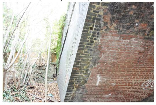
The horizontal spandrel crack is matched on the other side.
