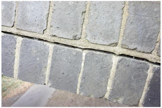
It is clearer on this side that there has been substantial repointing, but how long ago? And why was it confined to the lower three rings. Ahhh, as Hamish points out, three rings of new brick. Notice also the horizontal crack in the spandrel here. It must be related to backing level. Incidentally, that is a header in the ring just below the end of the crack.
