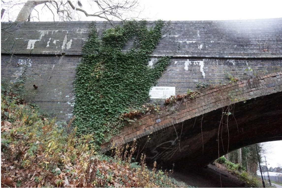
As at last month's bridge, there is a horizontal crack in the spandrel and some degree of ring separation near the end of it. Note the drain, which must come from the top of the backing, though the crack is below. The crack is quite substantial.
