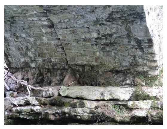
The first impression is of clay as though the stone facing has been lost. Luckily, I was able to go back to my previous set. Though I don't have a shot from this angle, the first image above can be pushed a little to reveal the condition from 2014.
