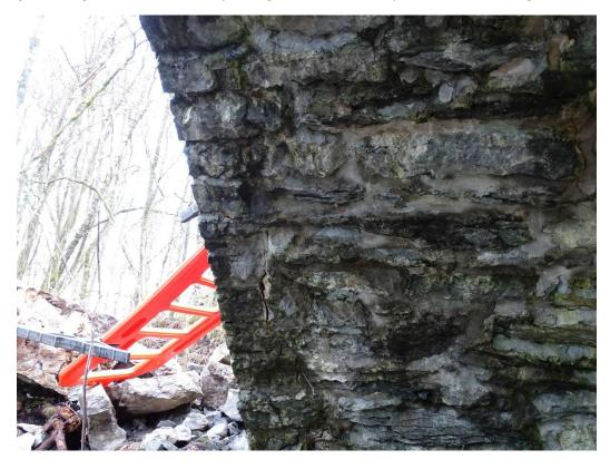
In the scale of things, this is modest damage and a sound rebuild job on the spandrel and parapet should improve matters.
