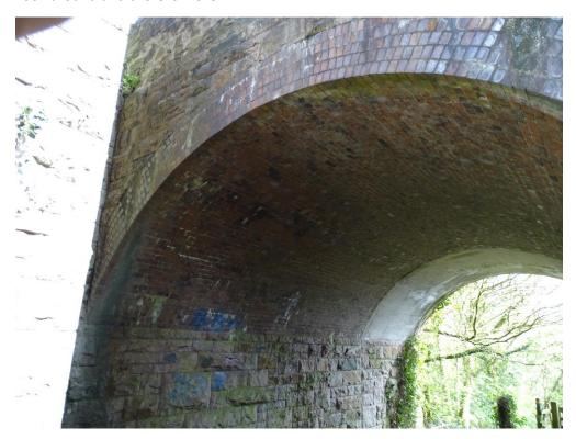
Brightly lit, to the left is the pier of the Railway viaduct. The arches (both brick and concrete) support the road.
