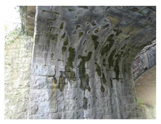
There has been a lot of mortar washed out, but the joints were thin and there has been little enough displacement of the stones. The extent of the string-course up there to the left is quite impressive. Look back to the one on last month's bridge, which was also a Brunel design. Both by the man himself or the same able assistant?
