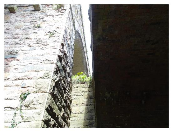
There is a retaining wall butting up against the railway pier, which is more clearly discerned here.
