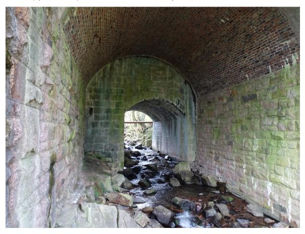
So, get back to the upstream side and we find that the other side of this older arch butts on to the viaduct pier.
