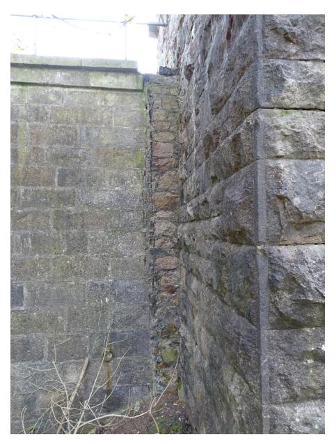
In the span where the path goes, there is a double wall. The perspective here doesn't show well, but the rear, rubble wall is the parapet of the present road and off the line of the viaduct and the dressed stone wall is the causeway approaching the stone arch of the old, much narrower road. Here we have two older versions of what is mow the A38 road to Plymouth. The newer one is a dual carriageway and runs about 300m away lower down the valley.
