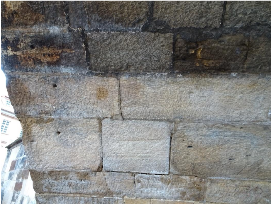
Looking closer, though those are surely modern scotch marks on the stone.
