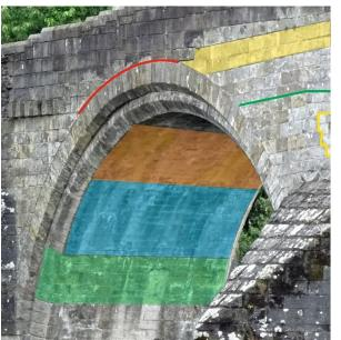
lowest of the coloured zones is very badly weathered. Above that is a band with dark water runs and above again, one with paler runs in distinct stripes. The lower band is very badly weathered, surely indicating considerable water penetration from behind.
