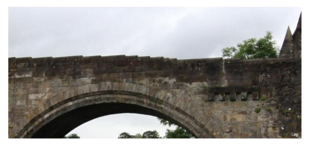
Looking more closely at the parapet and below on the upstream side there is a matching open joint round the top of the ring and extending along the bottom of the parapet. There is then a vertical crack in the parapet just above the corbels. There has been some form of settlement here, whether in the substructure or just the crown of the arch requires a closer investigation than I had time for.
