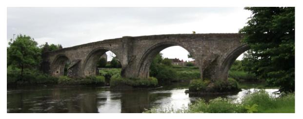
We know that one span was replaced in the  $17^{th}$  Century. I rather feel that the row of pigeon holes on the far pier here might be a sign of that later rebuild.
