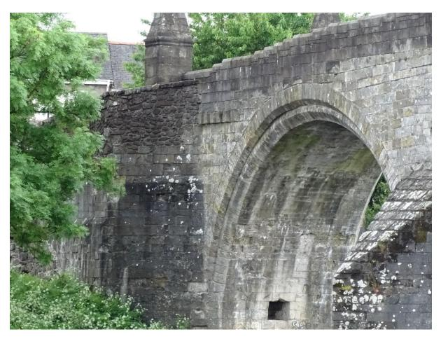
A similar set of corbels appears on the other side. It is understood there were once gates on the bridge. Perhaps these corbels mark the position. There are five different bands of condition in the visible half arch. Three are coloured in the view below but there is stone above and below too. The
