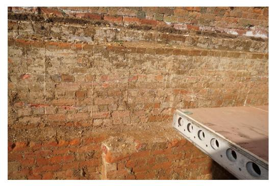
Looking in from the back end, note that the wing wall thickness steps in as shown on the original drawings.
