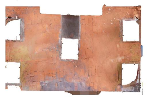
With the bridge lifted 900mm we were able to take enough photographs of the cut face in the north abutment to create a model and render a plan image. Unfortunately the surface (this is the top face) was not clean enough to show the bond near the edges. The windows are where the jacks were in position. The build of the bottom face was incomplete at the first attempt but we are working on that.
