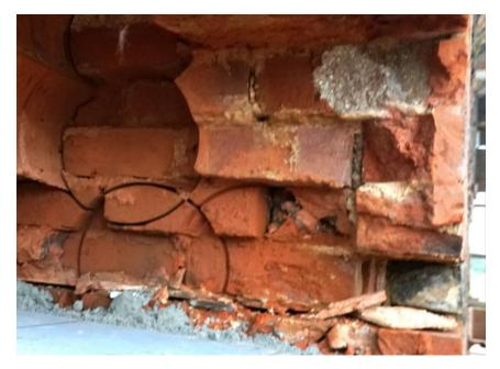
Here, the rubble packed into the header root is evident and the mortar in there very different from the original.
