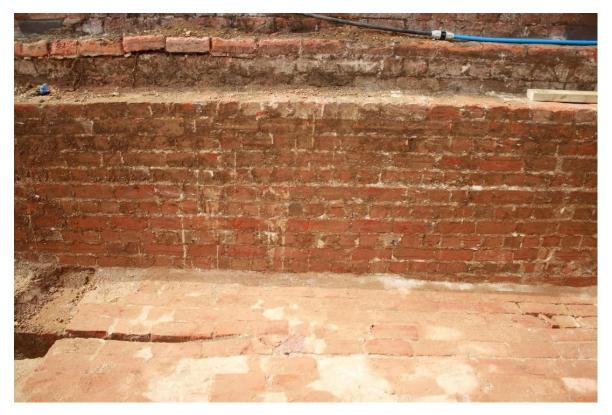
Looking to the side we can see that the courses in the upper wing wall are inclined (which means they match through thickness) whereas those of the backing are horizontal. This raises obvious questions about the bond between these two parts. Is it hit and miss, with a through brick wherever the courses lined up or is it just a butt joint?
