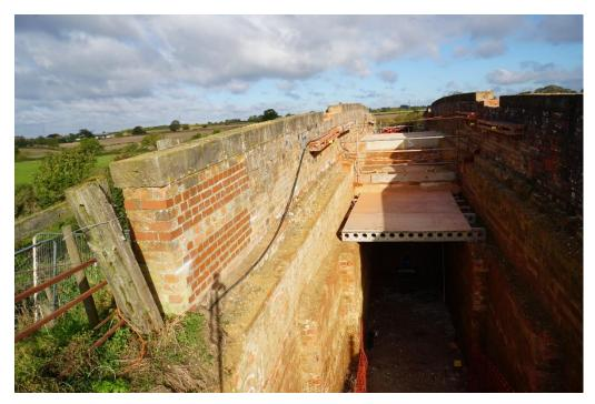
If you look back to the second picture you will see that the outer courses are horizontal at arch springing level and then progressively tilt backwards on very slightly tapered mortar beds. On the inside face, things are done more coarsely using bricks tipped up on edge to make steps. How and where the two meet remains unclear.
